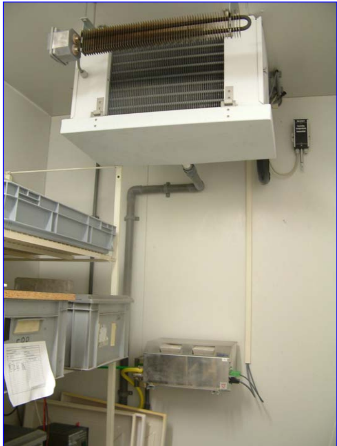
Material test bench of timber industry in the Netherlands.
